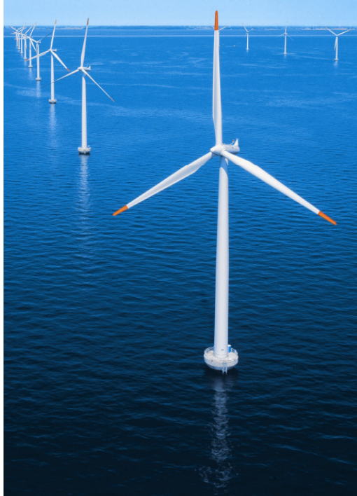
Abb.11: Windpark Nysted Siemens press picture
